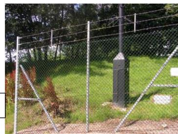
Picture 1 shows a standard BS 1722 Part 10<sup>13</sup> chain link fence, approximately 2.9m high constructed with chain link fabric and a barbed wired topping. Supporting posts can be either reinforced concrete or tubular steel.
