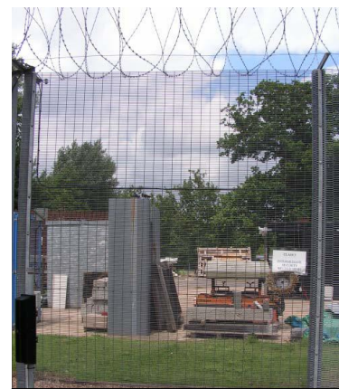
Picture 3: Class 3 security fencing
